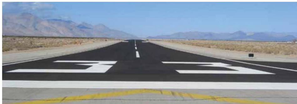
Figure 10. Reinforced runway overlay at Inyokern Airport, California (Mojave Desert) [3].
