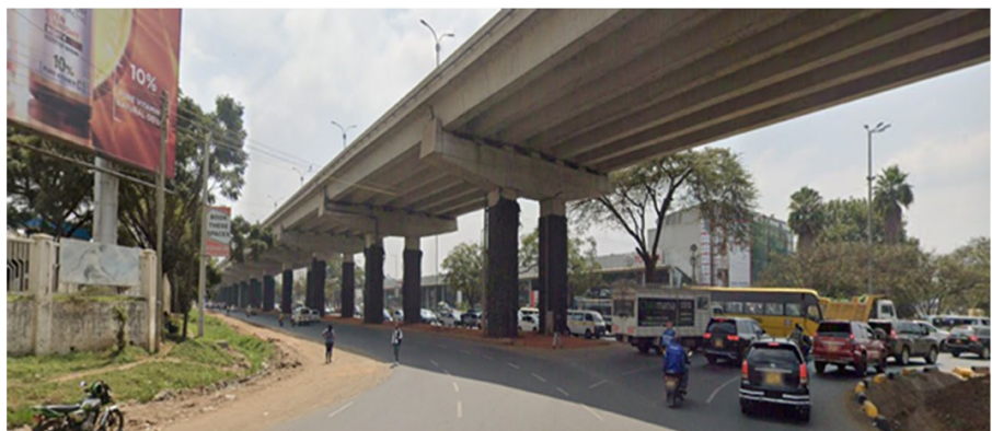
Figure 18. Street view of Uhuru Highway.
