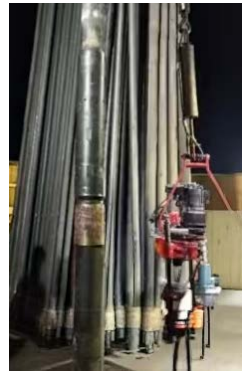
Figure 6. Photographs of drill-free glass blind plate valve running into the well and pressure-induced crushing.
