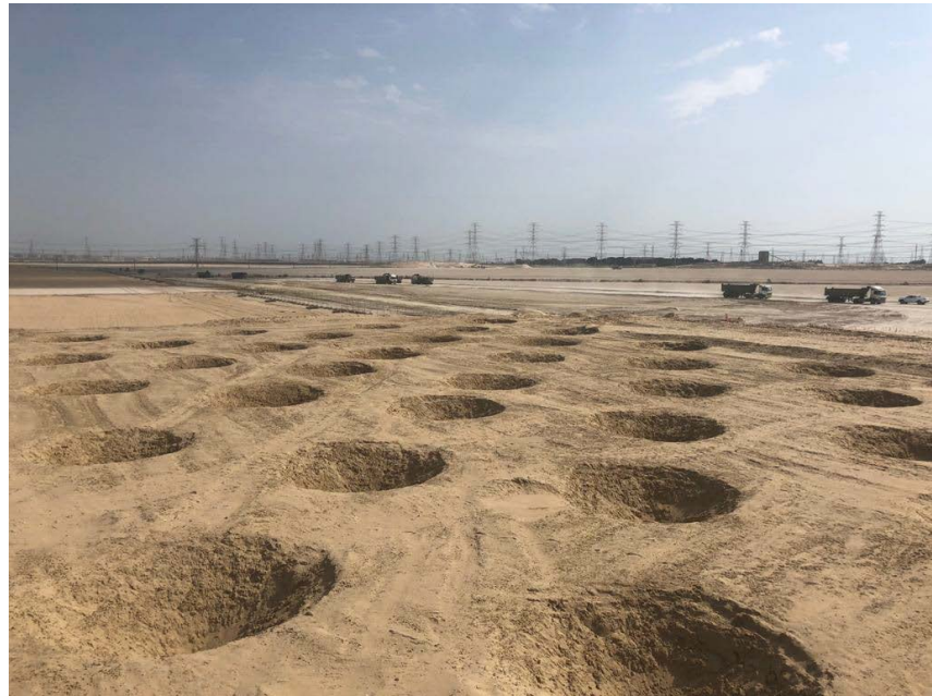
Figure 3. Post dynamic replacement craters after application.
