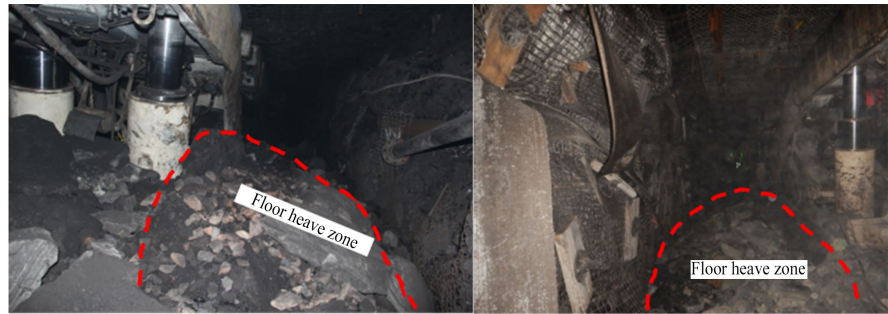
Figure 13. Comparison of tail bottom drum before and after hydraulic fracturing.
