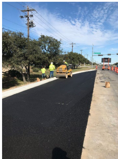
Photo 11. Executing pavement construction activity.
