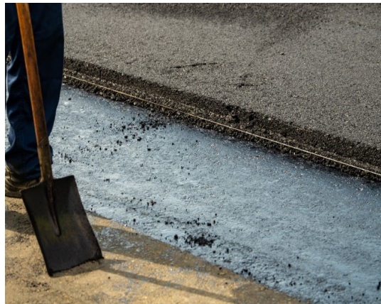
Photo 14. FRAC 70 mm thick surface course layer.
