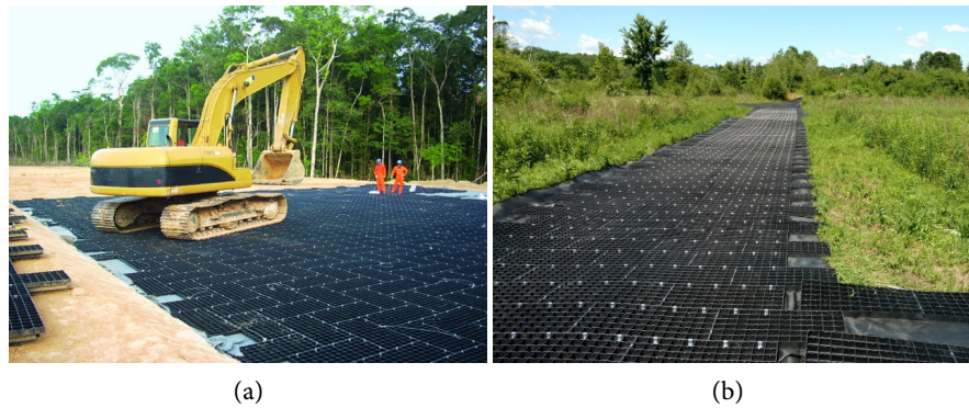
Figure 6. Site lay-down areas and access road [24].
