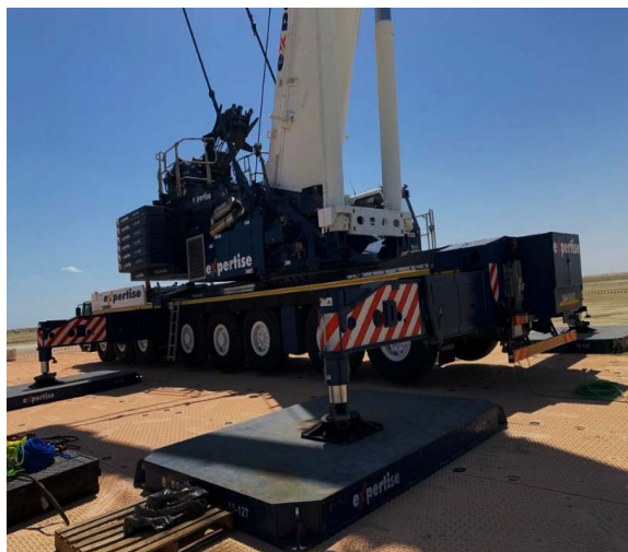
Figure 12. Positioned crane on top of the laid GAM [29].
