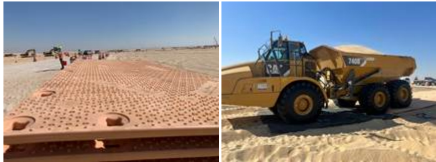
Figure 15. Mat application at SPARK construction site [29].
