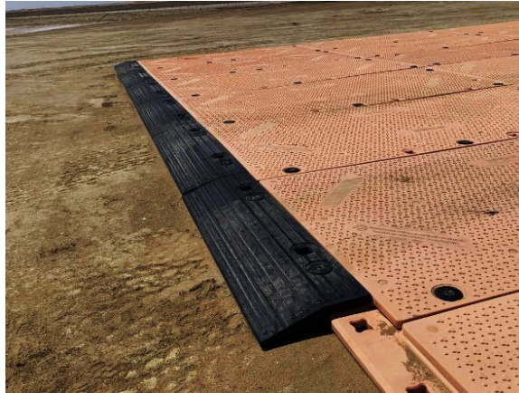
Figure 11. GAM laid on ground and supplied with a ramp [29].
