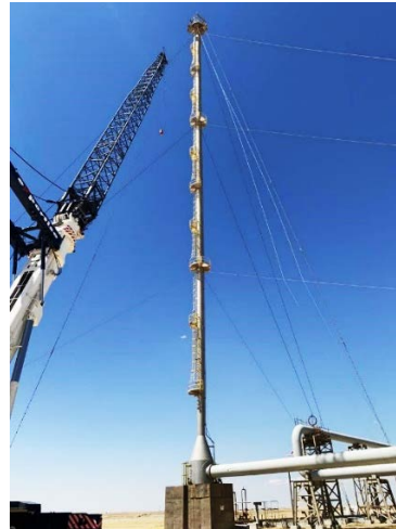
Figure 13. A crane performing the lifting supported by the GAM [29].
