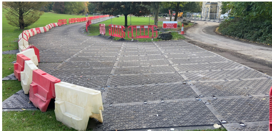
Figure 5. Temporary access road [23].
