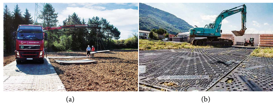
Figure 9. Temporary access road in poor/water logged soil [27].
