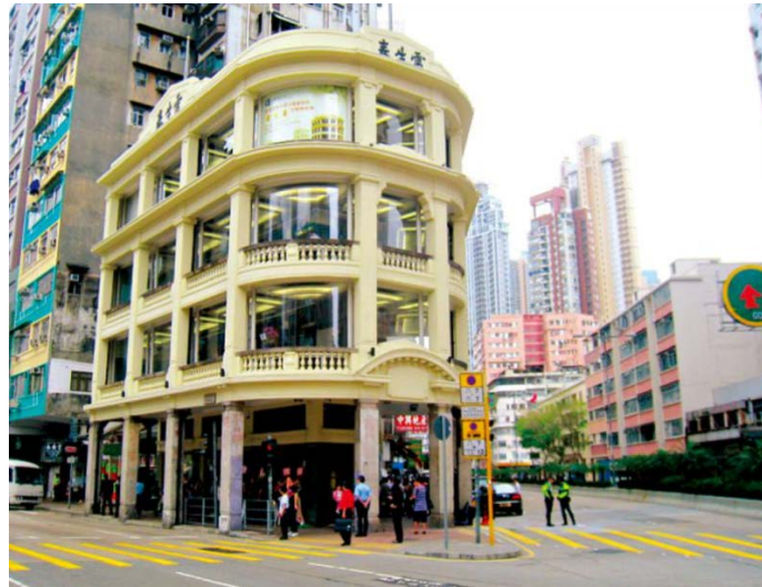
Figure 4. Qilou buildings in Hong Kong.
