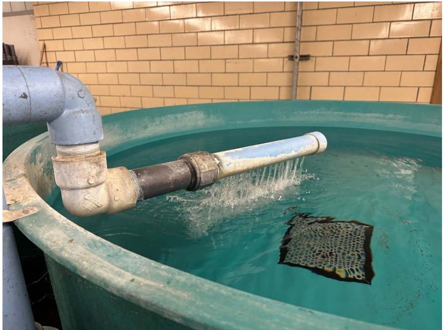
Figure 1. Image of an elevated spray bar in a 1.8-m diameter circular rearing tank.
