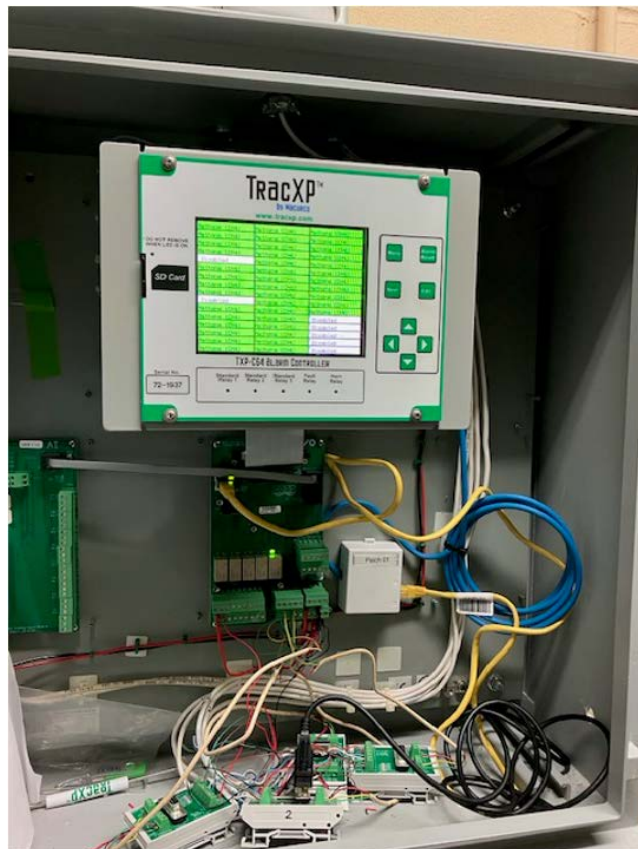
Figure 15. Controller system display after installation and troubleshooting were completed (Note: Grey spaces represent empty channels).
