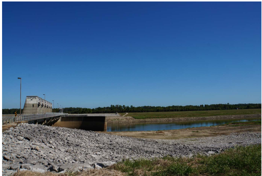
Figure 33. Old river control complex spillway.
