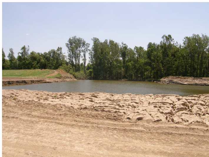
Figure 26. Breached New Madrid floodway levee at Birds Point. Photograph taken by Lois Wright Morton.
