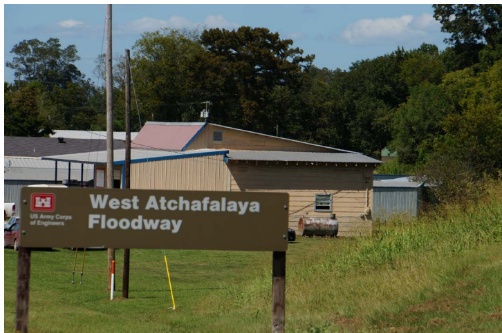
Figure 42. West Atchafalaya floodway sign with protected structures and levee in background.
