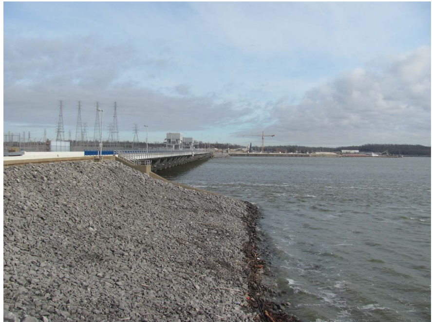
Figure 36. Wide Kentucky dam and reservoir.
