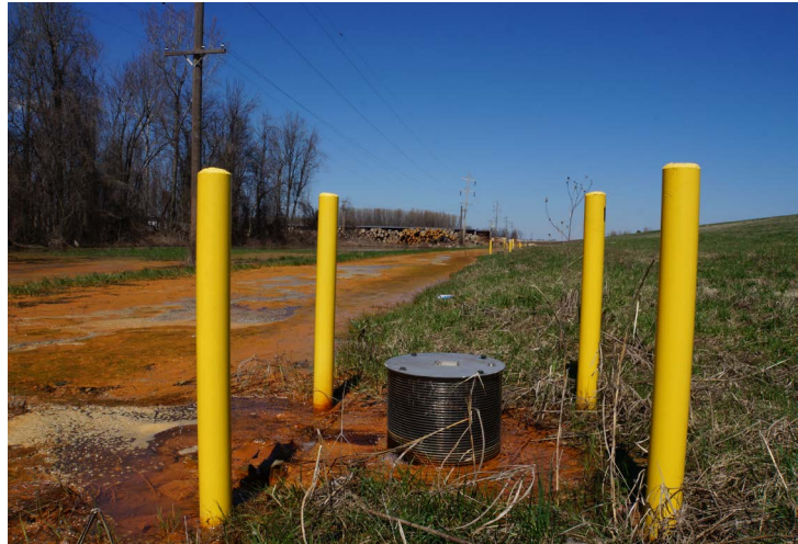
Figure 30. Relief well along the Ohio River and Levee Street. Published with copyright permission from Book Editor of Soil and Water Conservation Society.
