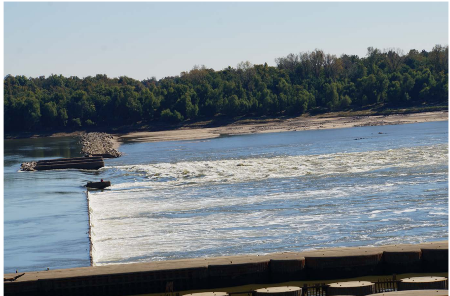
Figure 49. Dikes and dams on the Lower Mississippi River and tributaries.
