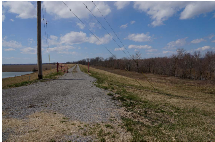
Figure 41. The Little River drainage district diversion embankment. Published with copyright permission from Book Editor of Soil and Water Conservation Society.
