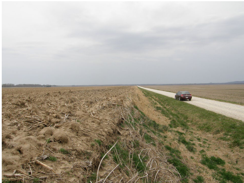
Figure 11. A filled Sny River settling basin that is 3 m above the land surface. Reprinted with permission from the Editor of the Journal of Soil and Water Conservation.
