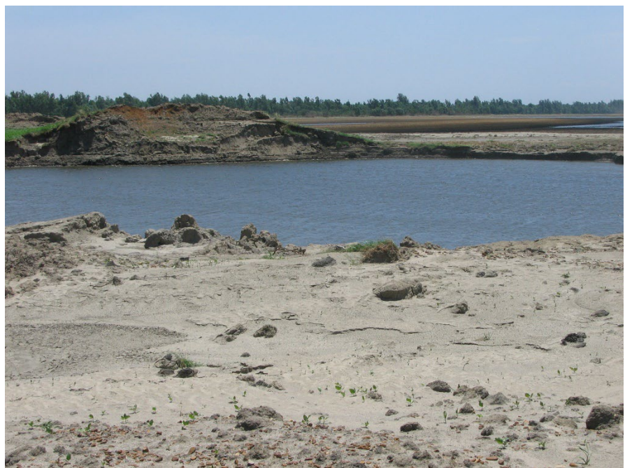
Figure 17. The Birds Point levee was the site of the first explosion on May 2, 2011, that opened the New Madrid Floodway and relieved river pressure on the Cairo floodwall. Remnants of the fuse plug levee and the crater lake extend into the adjacent agricultural lands. Photo Credit: Lois Wright Morton. Reprinted with permission from Editor of Journal of Soil and Water Conservation.
