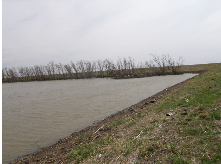
Figure 9. The Pigeon Creek settling basin west of Hull, Illinois, is currently active during high runoff and flooding. Reprinted with permission from the Editor of the Journal of Soil and Water Conservation.
