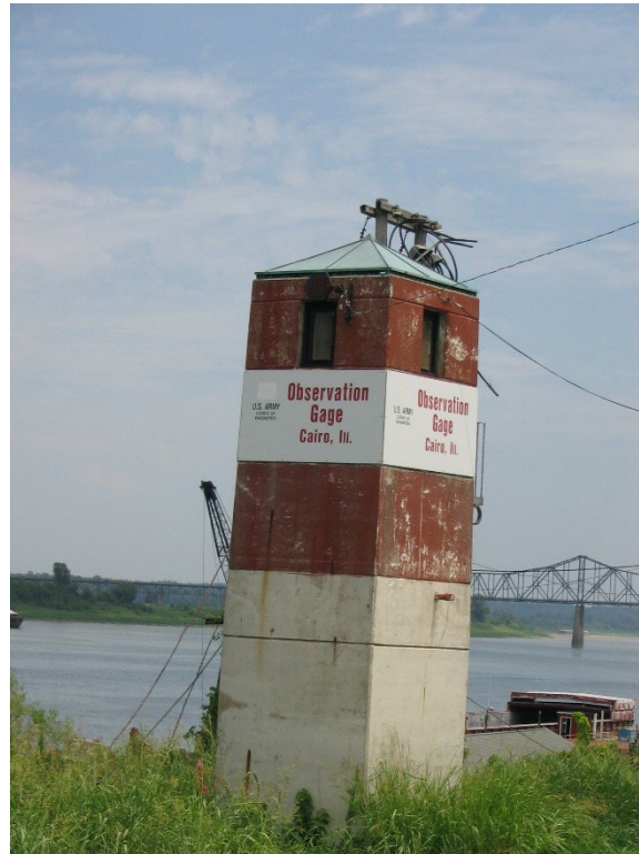
Figure 3. The Cairo, Illinois, river gage on the Ohio River is used to determine river height and when it is necessary to open the Birds Point–New Madrid Floodway to relieve downstream river pressure. Photo Credit: Lois Wright Morton. Reprinted with permission from Editor of Journal of Soil and Water Conservation.
