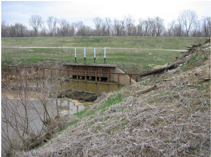
Figure 6. The Sny River aqueduct passes under the Kiser Creek Diversion channel. Reprinted with permission from Editor of Journal of Soil and Water Conservation.
