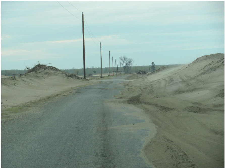
Figure 29. Mississippi River floodwaters deposited many tons of sand on farmland and roads in Dogtooth Bend peninsula when the Len Small levee breached in January of 2016. The sand dunes left behind required graders and snowplows to open the road for local traffic. Reprinted with permission from Editor of Journal of Soil and Water Conservation.
