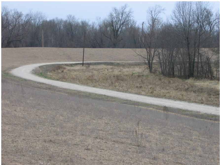
Figure 8. The merged Mississippi River and Kiser Creek Diversion levee blocks the Sny River channel flow, and water has to be pumped over the levee to the Mississippi River. Reprinted with permission from the Editor of the Journal of Soil and Water Conservation.
