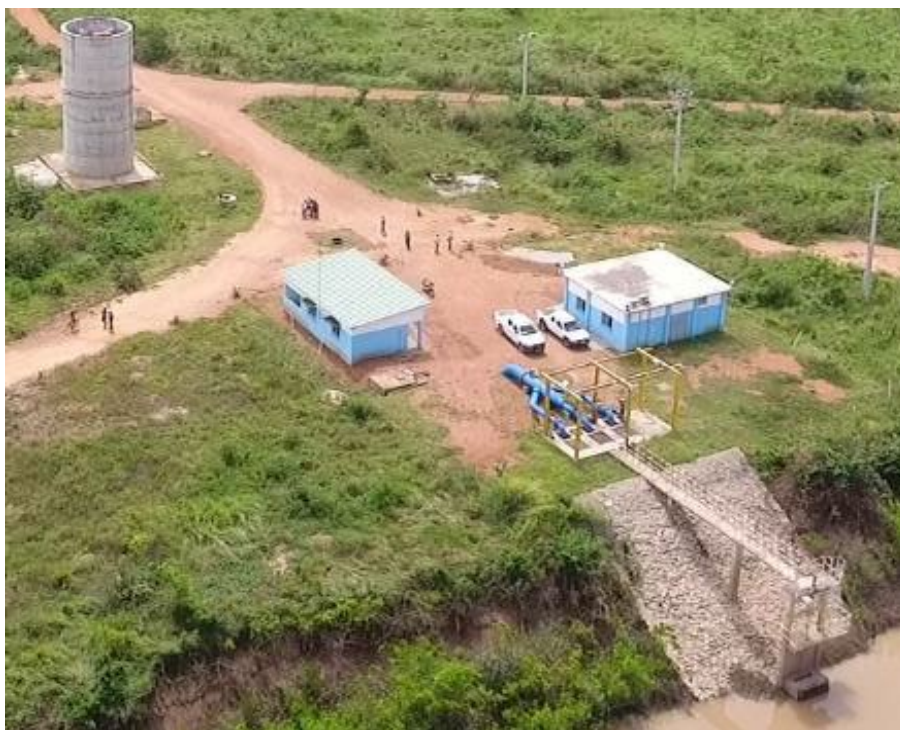
Figure 2. First water pumping station in the M'Bahiakro irrigated area.
