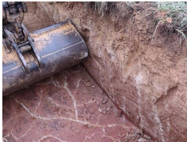
Figure 1. An exposed fragipan soil showing the inter-prismatic gray veins that separate the consolidated impermeable prism areas.
