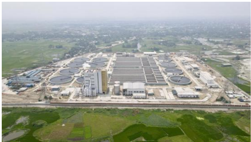
Figure 27. The largest sewage treatment plant on the Ganges-Brahmaputra rivers in Bangladesh.
