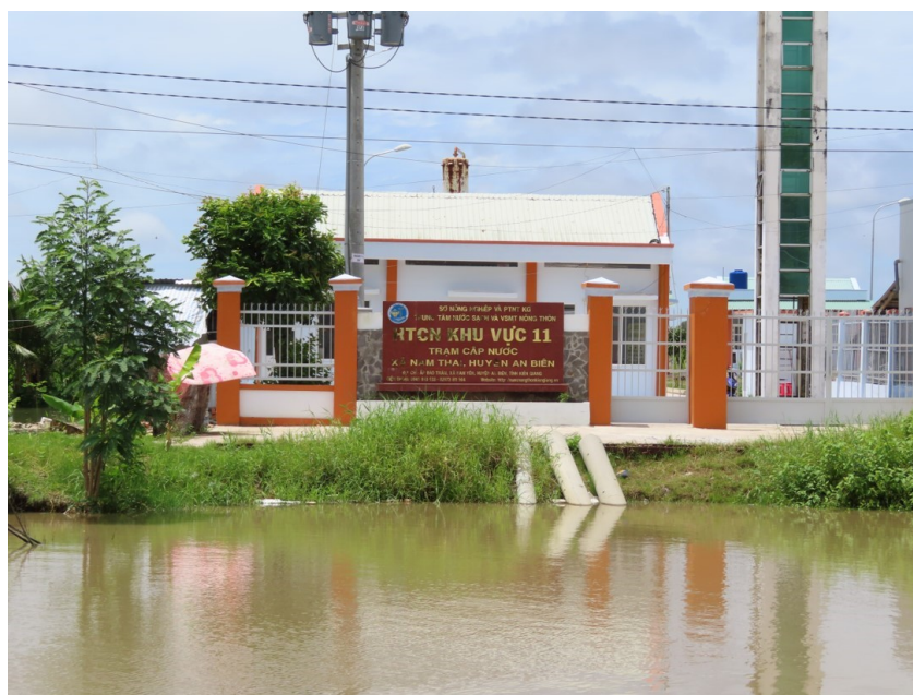
Figure 25. A water treatment plant in SE Asia. Published with permission of the Editor of Open Journal of Soil Science.
