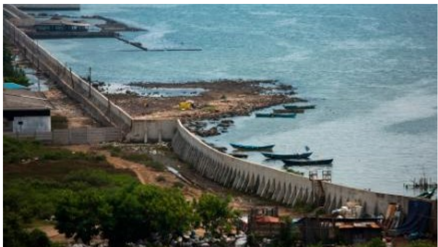
Figure 13. Jakarta floodwall. Published with permission of the Editor of Open Journal of Soil Science.
