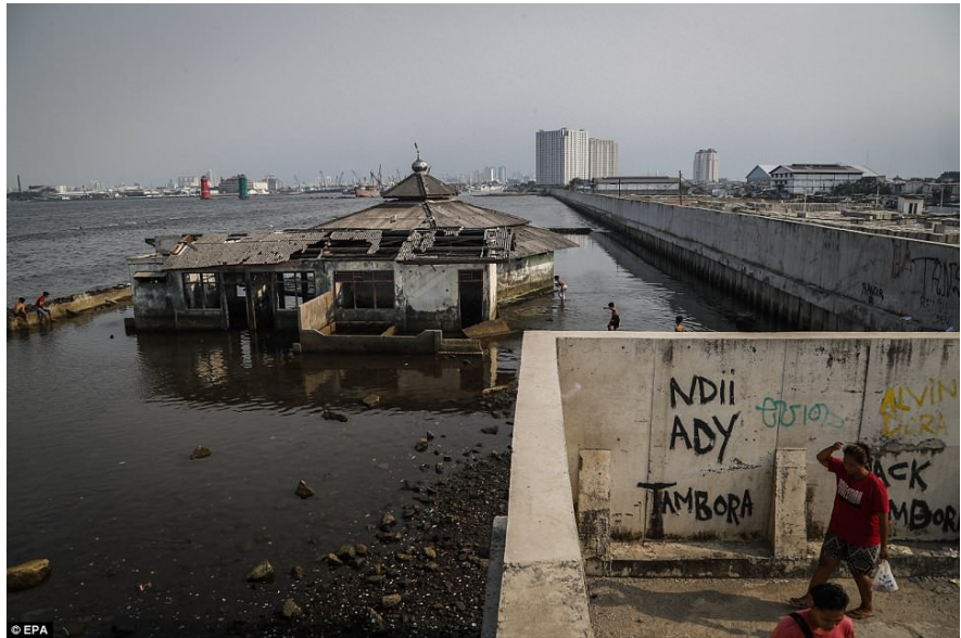
Figure 14. Close-up of Jakarta floodwall insert. Published with permission of the Editor of Open Journal of Soil Science.
