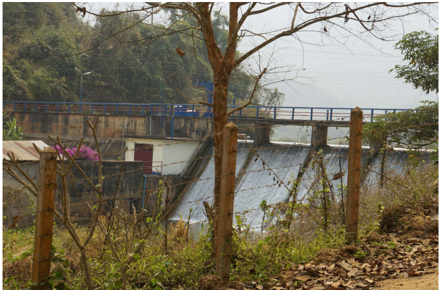
Figure 30. Hydroelectric power is produced from a small dam on a Mekong River tributary in the northern Lao People's Democratic Republic highlands. The reservoir behind the dams is used as a fishery and for irrigation. Published with the permission of the Editor of Open Journal of Soil Science.
