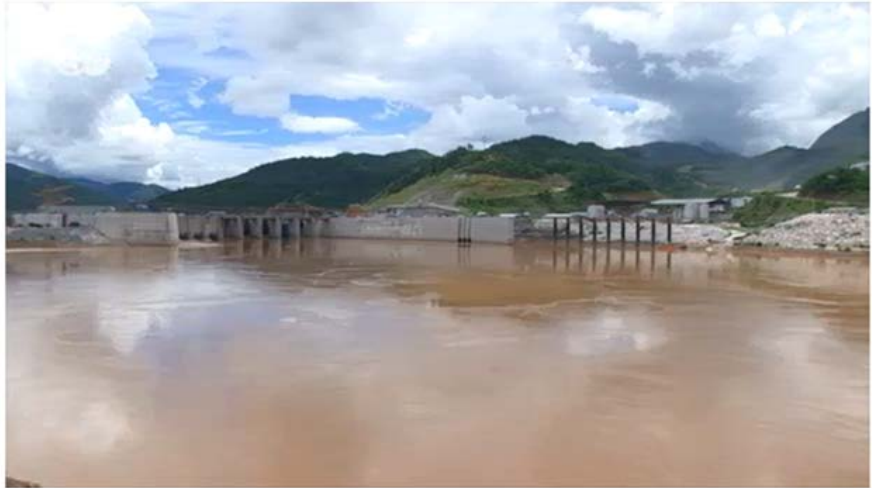
Figure 32. Xayaburi dam in Laos. Photo Credit: Mekongeye.
