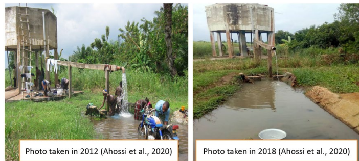
Photo 1. Photos showing the flow rate of an artesian borehole tapping the aquifer in 2012 and 2018.
