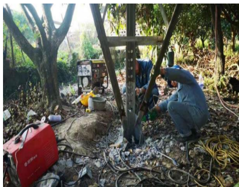
Figure 3. Main pole replacement.
