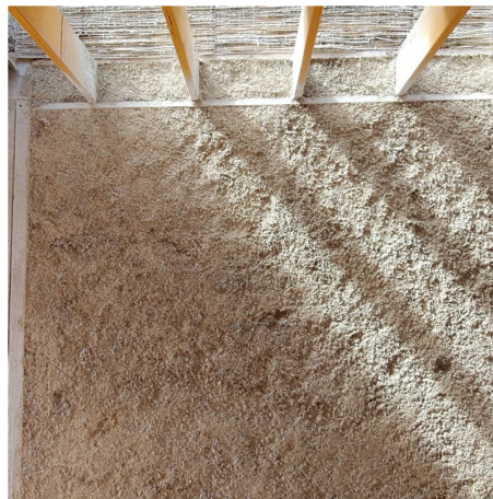
Figure 12. Hempcrete wall insulation ( https://hempstone.net ; used with permission).
