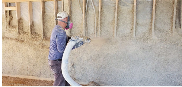
Figure 10. Spaying hempcrete on the wall ( https://hempstone.net ; used with permission).
