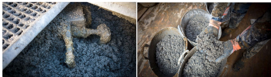
(a) Hempcrete during mixing process
