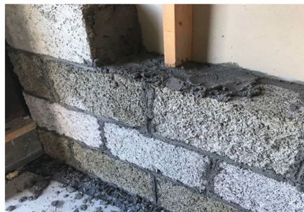
(b) Block mortar made with hempcrete binder + masonry sand
