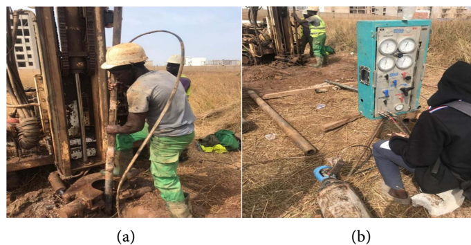
Figure 4. Core drilling and pressuremeter testing.
