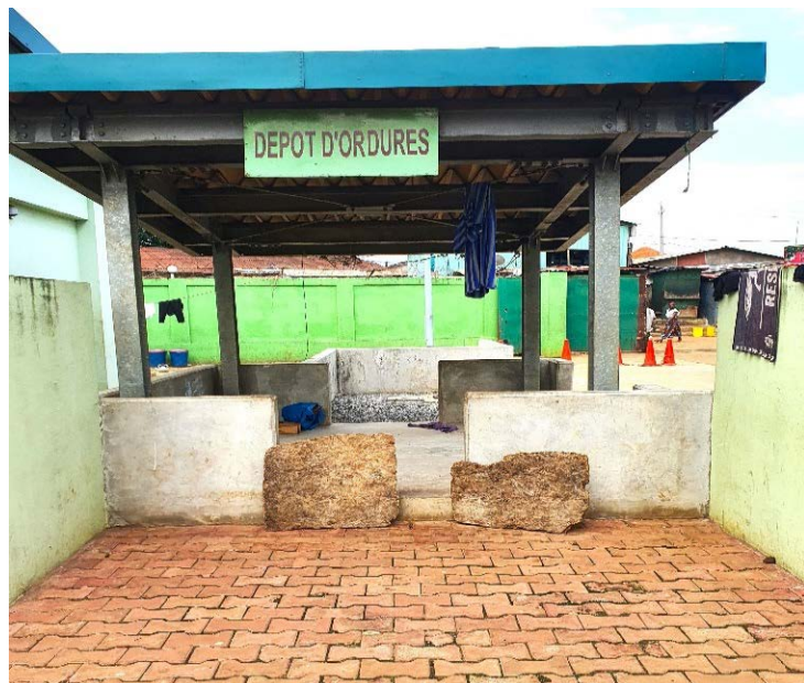
Figure 4. Showing the shed designated for waste disposal.
