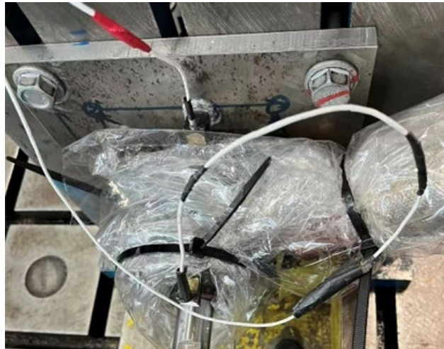
Figure 3. Air-heating/air-cooling temperature control system.
