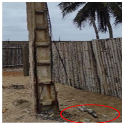
Figure 10. Concrete spalling.
