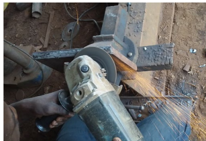
Figure 7. Cutting the sheets.
