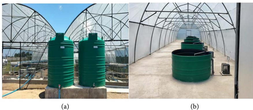
Figure 4. Images of water tanks in Port Durnford (City of uMhlathuze). Source: Fieldwork (2024).
