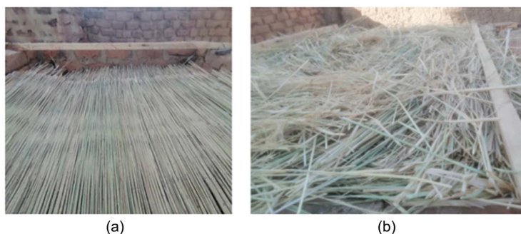
Figure 6. Roof Insulation: (a) Installation of reed mats on the underside of the roof; (b) Distribution of rice straw (sample 4).
