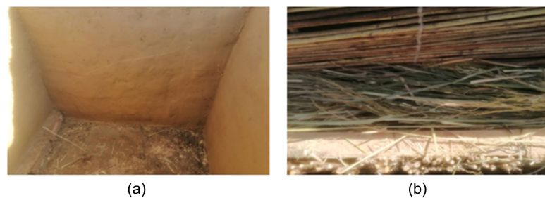
Figure 5. (a) walls coated with a raw clay plaster; (b) rice straw placed between two reed mat walls (sample 2).
