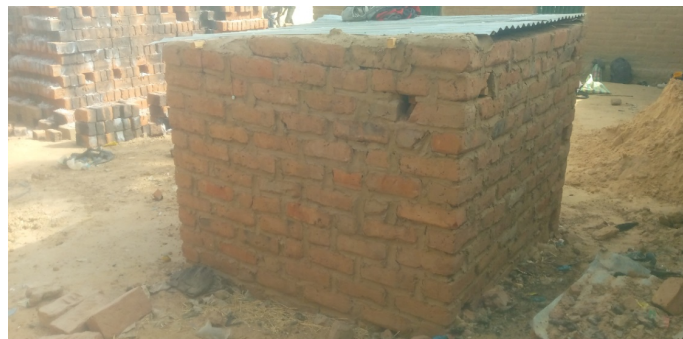
Figure 3. Experimental cell constructed as part of our study.
