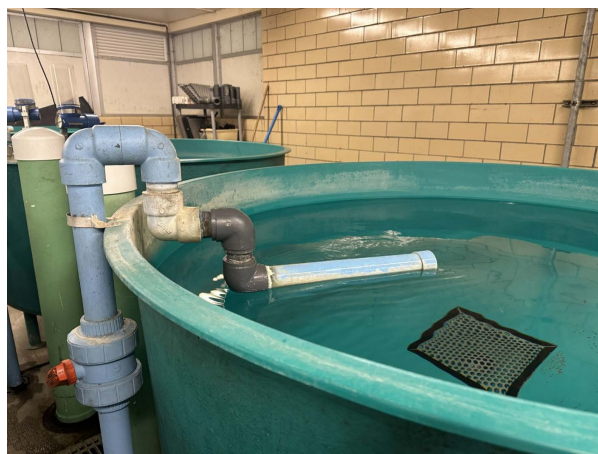
Figure 2. Image of a submerged spray bar in a 1.8-m diameter circular rearing tank.
