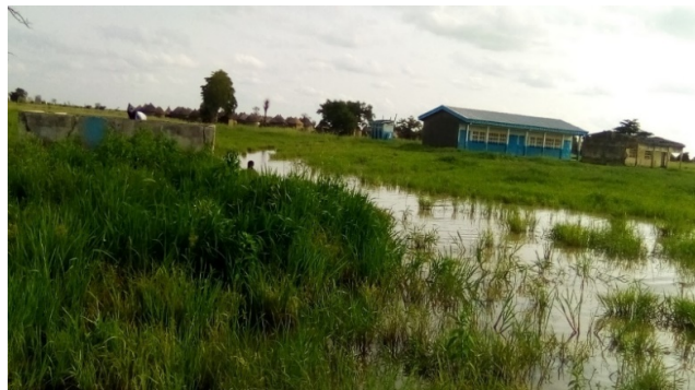
Figure 6. Flooding of a residential area in the Waidoua neighbourhood (Vele).
