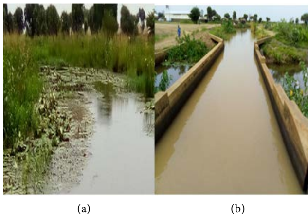
Figure 8. Main channels: drainage channel (a) and irrigation channel (b) of SEMRY.
