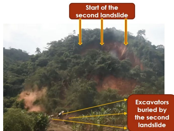
Figure 3. Starting of the second landslide.
