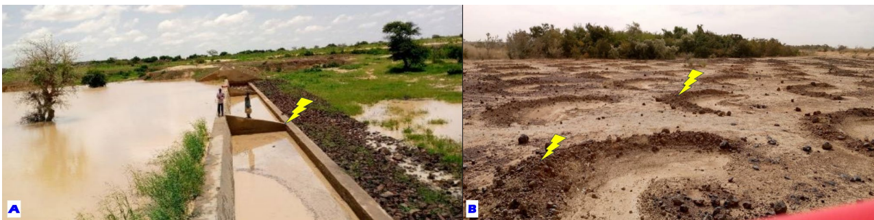
Figure 14. Sustainable water and land management techniques in the sub-basin: (A) Awa Data spreading weir and (B) half-moon fields on the banks (Zango 2025).
