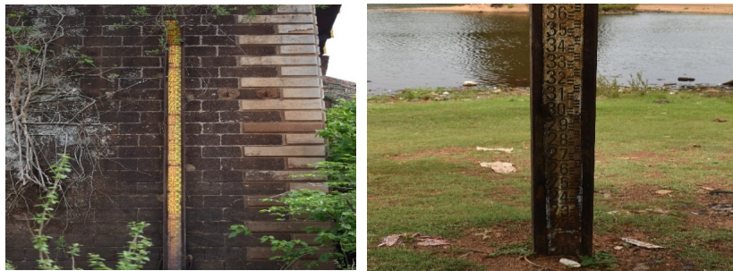
Figure 1. Enamelled steel sheet water level gauge installed at the foot of the historic bridge and in the riverbed in the urban commune of Kouroussa.
