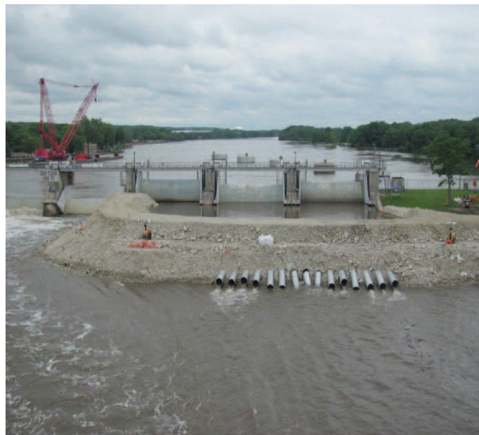
Figure 11. Temporary dike and pond created below the 3 damaged gates on the Marseilles Dam [2].
