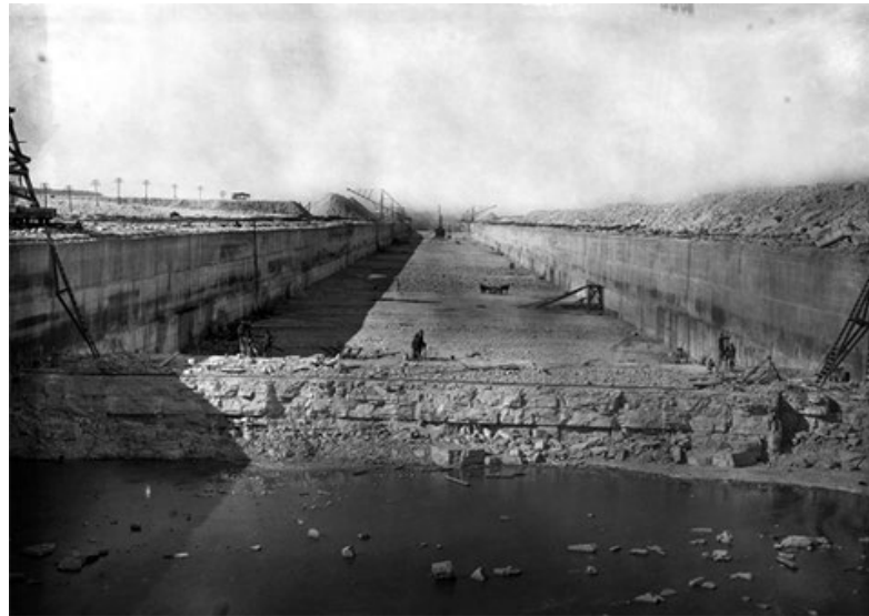
Figure 3. Chicago Sanitary Canal used to reverse the flow of the Chicago River and to transfer sewage from the Great Lakes drainage basin to the Mississippi River drainage basin [7].
