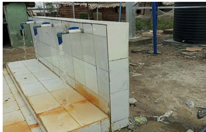
Figure 7. Reddish-brown color stain on water fetching platform showing high Fe content in the water.
