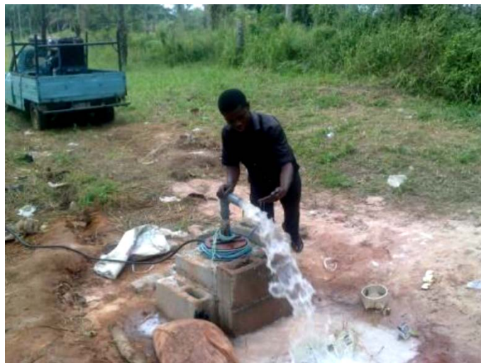
Figure 6. Observed high borehole yield in Azama Community during rapid pumping test.
