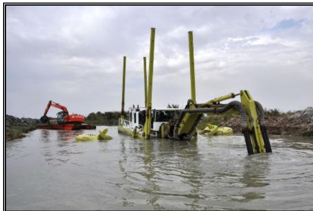
Figure 3. A dredger of type backhoe working on Tigris River (source [8]).
