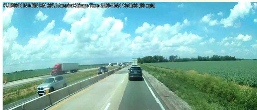
Figure 10. Dash camera image along I-65 in Indiana showing pavement marking and shoulder inconsistencies.
