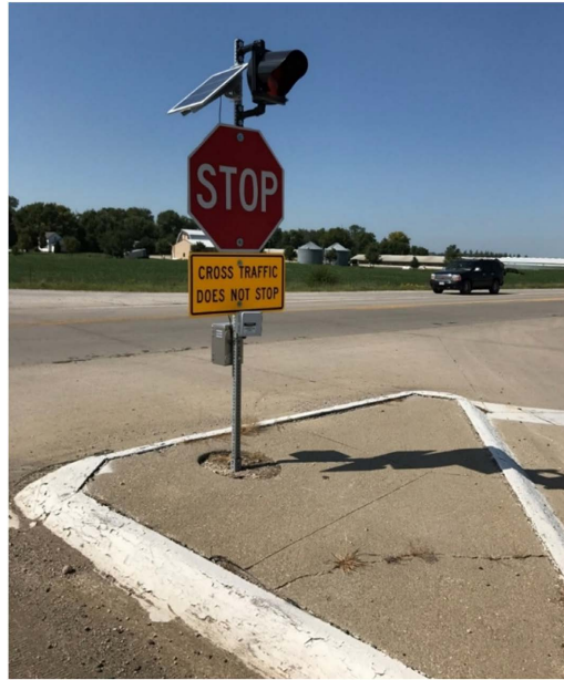
Figure 1. Flashing beacon installation.
