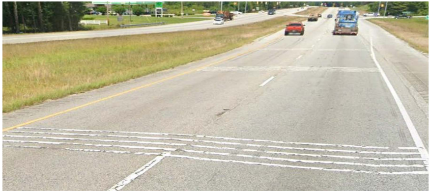
Figure 6. Transverse rumble strip (horizontal white lines) at US-280 & Grand National Parkway in Auburn, Alabama.
