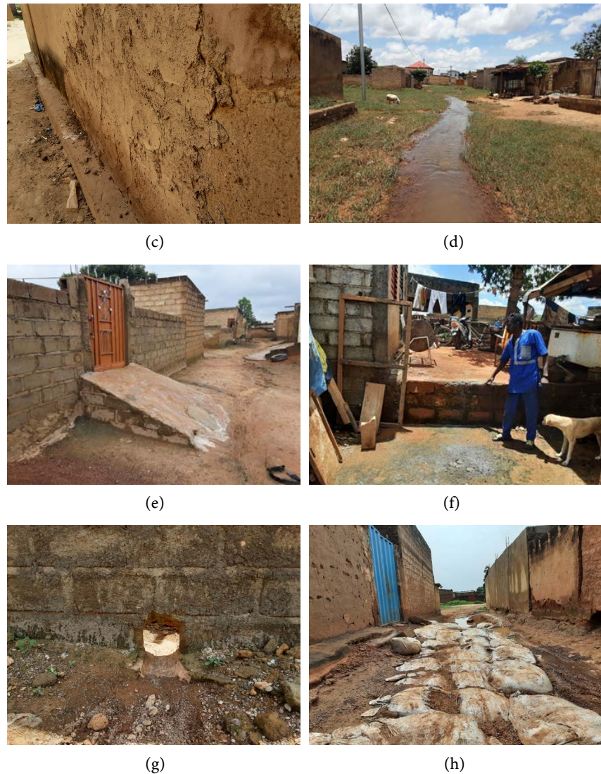
Figure 3. Illustrations of preventive flood protection measures implemented by different households: (a) Solid construction; (b) and (c) Protection belt; (d) Installation of trenches/ditches; (e) Raising the door threshold; (f) Elevation of housing; (g) Perforation of fences; (h) Placing sandbags.
