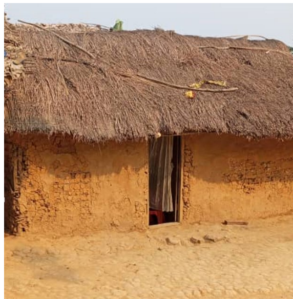
Figure 6. The most typical house type; huts with clay walls and thatched roofs.
