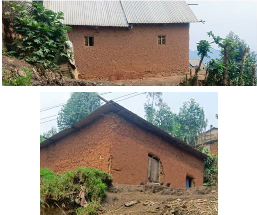
Figure 14. Mud and iron-sheet roof houses.
