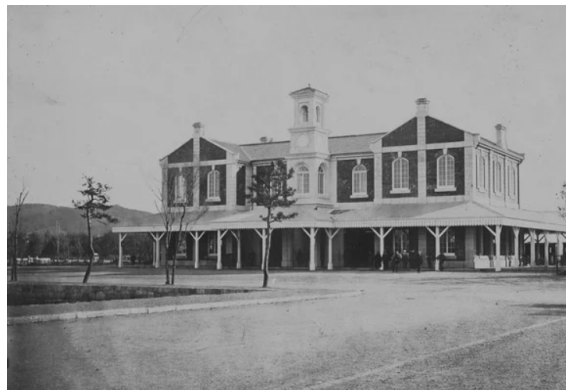
(a) Kyoto Station in 1914s
