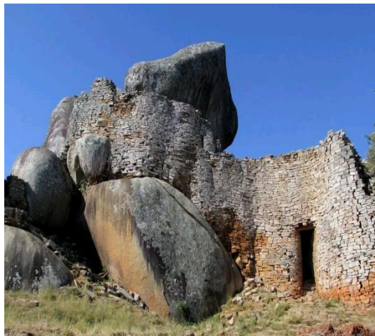
Figure 6. P-style stone wall on granite boulder foundation. Source: PBS learning media.
