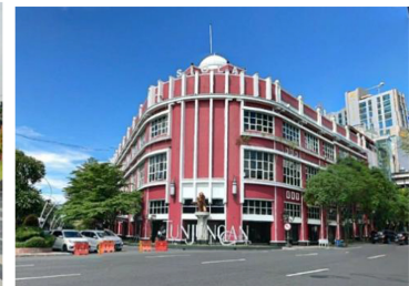
(c) Siola Building (Unair, 2023b)
