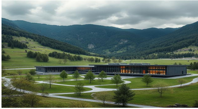
Figure 7. Elementary school complex, AI generated.
