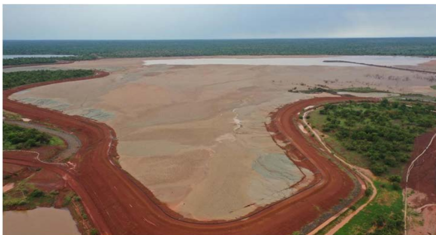
Figure 2. Aerial view of the Sabodala tailings storage facility.
