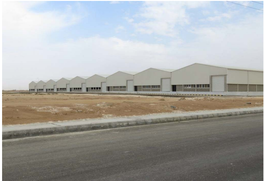
Figure 4. A sample of a ready hangar available for leasing in the industrial area of Mafrag (Adapted from reference 24).
