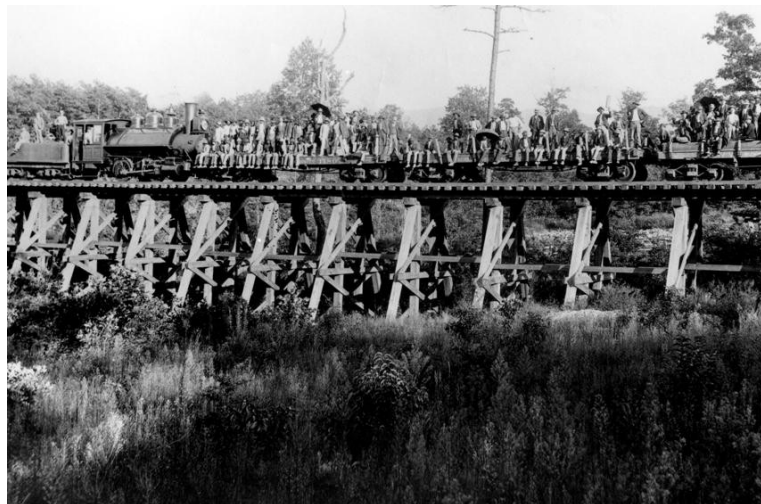
Figure 4. Train used to bring materials and visitors to Biltmore House.
