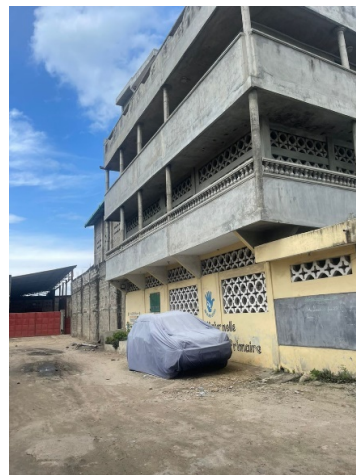
Figure 3. Car protected against cement dust.
