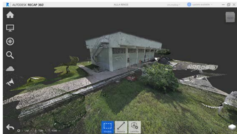
Figure 10. Point cloud of Renewable Energy Laboratory building from photographs with a mobile phone camera (Source: Authors).
