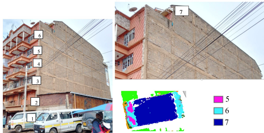
Figure 12. (a) shows a sampled building with both front and side view Figure 12(b) the zoomed building on the side view section of Figure 12(a) shows extra floor, Figure 12(c) shows the estimated floor numbers from the drone.
