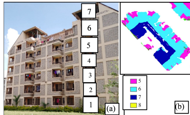
Figure 8. (a) Photo showing building with water tanks provision, (b) floor numbers as captured by drone data representing the building.
