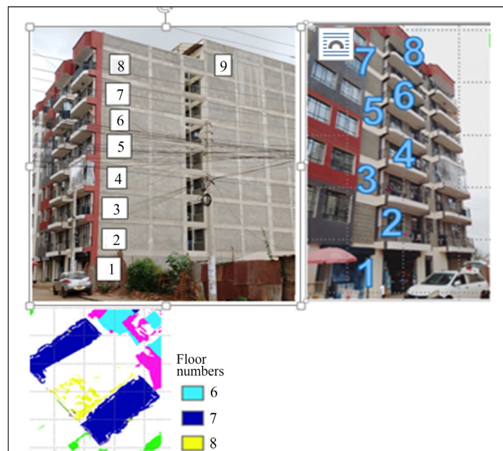
Figure 11. (a) Side view of the building, (b) front view of the building, (c) floor numbers as estimated from the drone data.
